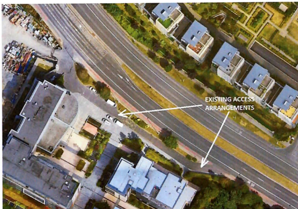
Figure 3: The Grange, existing access arrangements
