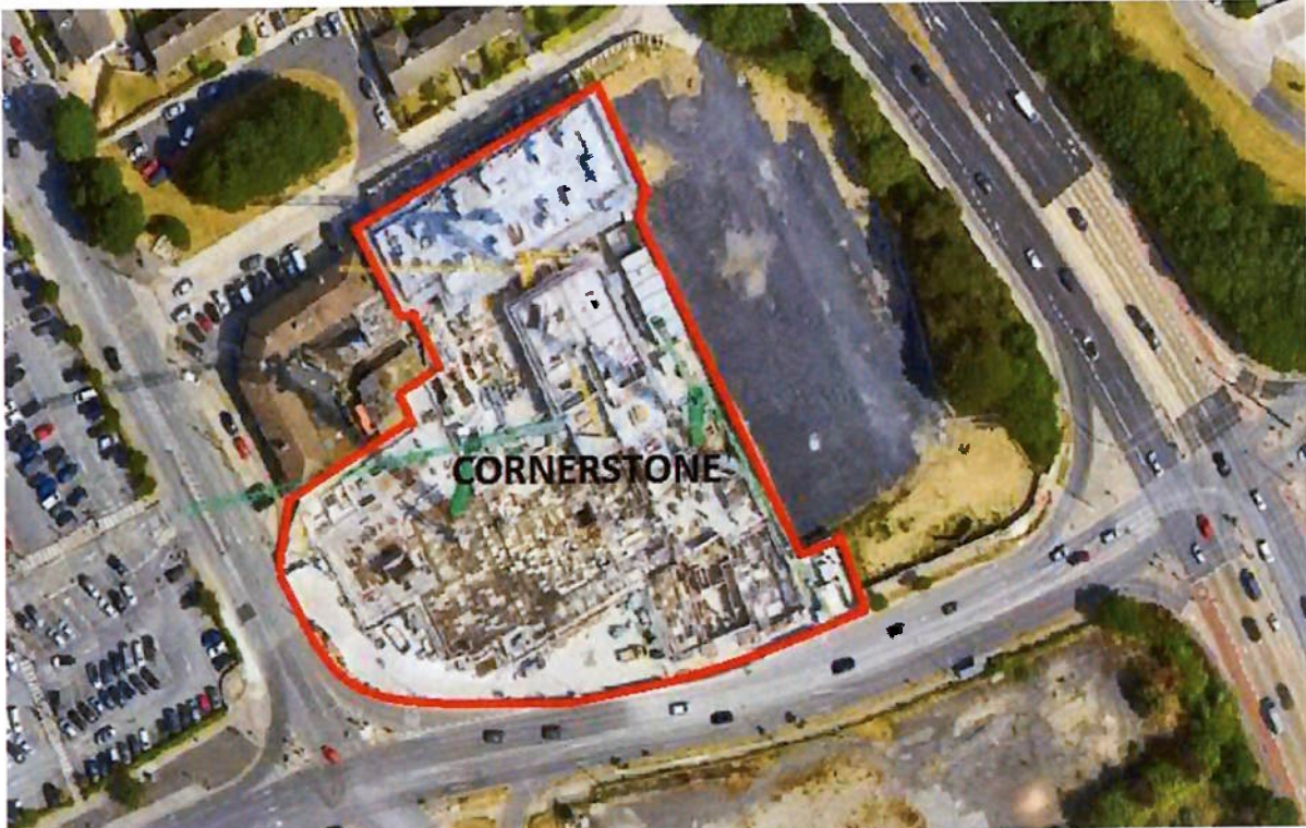
Figure 2: Comerstone (former Leisureplex site), Lower Kilmacud Road, Stillorgan
